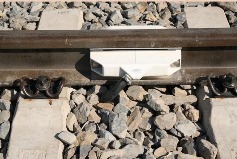
Axle counter, to keep safe distances between trains
